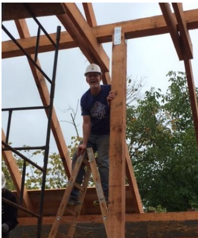
JO working on the house trusses
